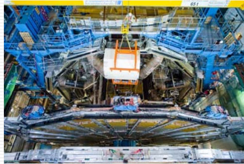
Installation of Inner Detector End-Cap
