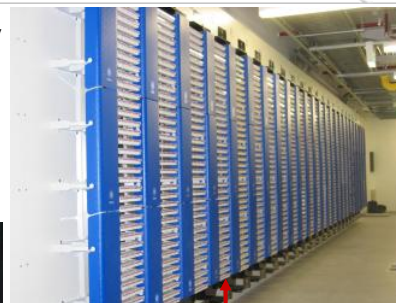
Wall-mount Cat 6 A Distribution Frame
